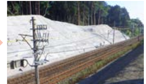
After the measures were carried out
