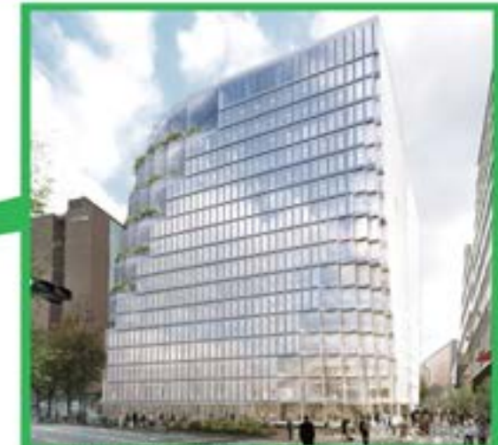
Tenjin Business Center Project (provisional name)
