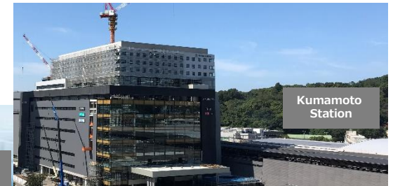
Status of construction of Amu Plaza Kumamoto (photographed on September 29)
