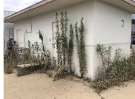
Equipment room flooding above the floor level
