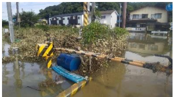
Damage to crossing equipment due to flooding
