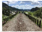
Rails from the track were cut and driven into the ground as earth retaining piles for the dedicated road, and the ballast was mixed with gravel and reused as a base for the pavement. 42
