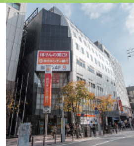
Tenjin Nishi-Dori Center Building
