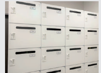
Installation of personal lockers
