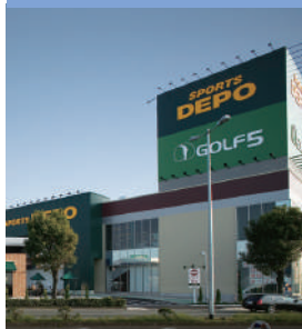
Kumamoto Intercommunity SC
