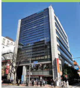
Sanix Hakata Building
